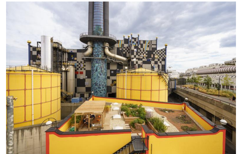
Power to heat plant Spittelau (10 MW)
